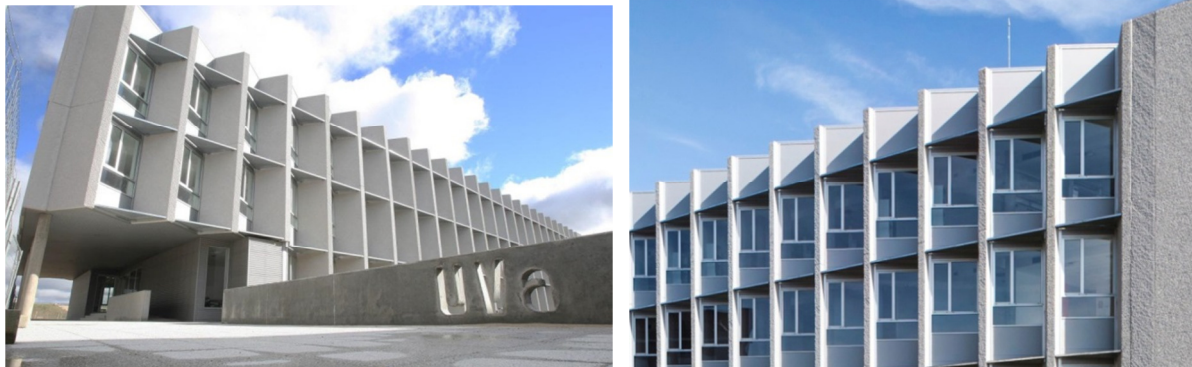
Fig. 1- Optimized compactness- South- West façade. Fig.2 Zig-zag façade to obtain self-shadowing effect.
