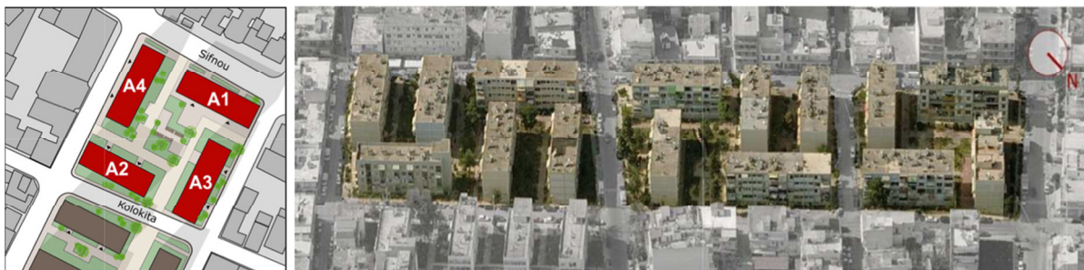
Image 1. Aerial View of Agia Varvara. In the three blocks are located fifteen buildings oriented according to the North-South and East-West directions. The classification among the buildings: oriented along the East-West direction with the living areas facing North (A1), oriented along the East-West direction with the living areas facing South (A2), oriented along the North-South direction with the living areas facing West (A3), oriented along the North-South direction with the living areas facing East (A4).
