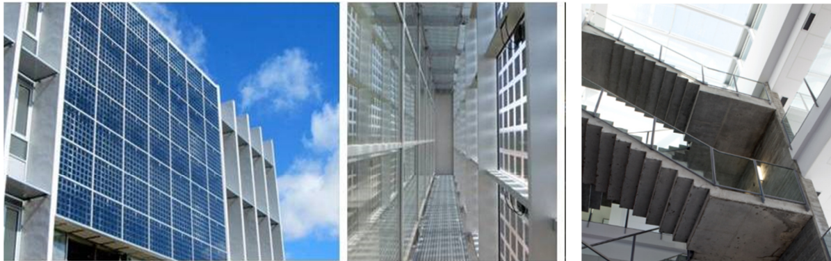
Fig. 7 and 8- Integration in façade of double skin curtain wall (External and internal). Fig 9- skylights above the staircase
